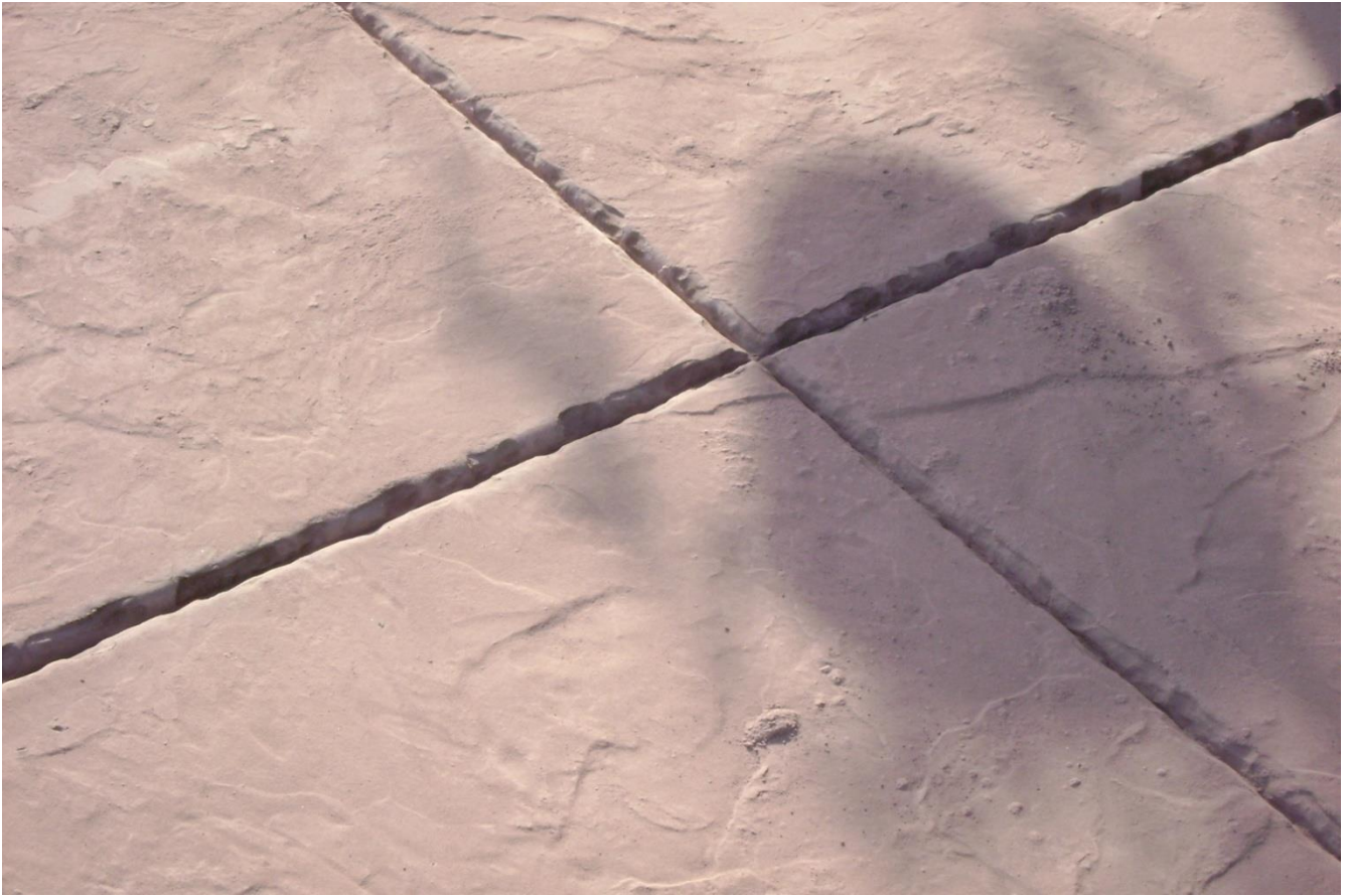
The photograph above is a hammered edge concrete path.
